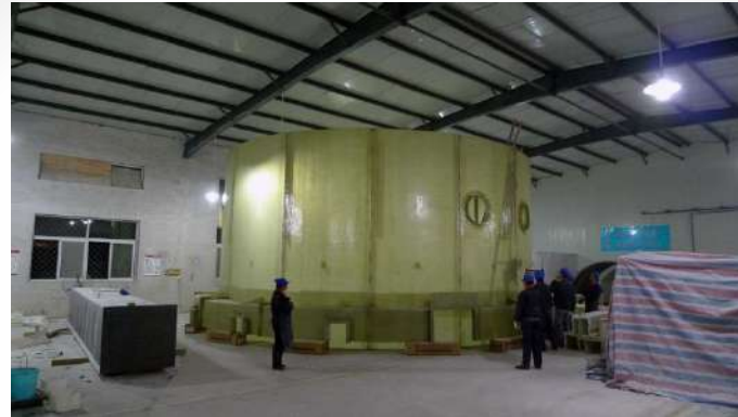
Reaction wells for 85' dia. clarifiers
