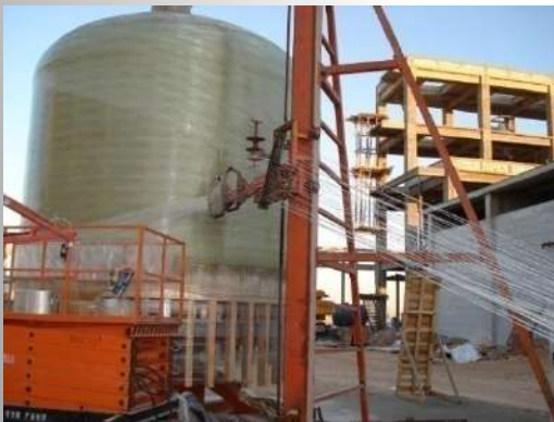
Field winding of large tanks
