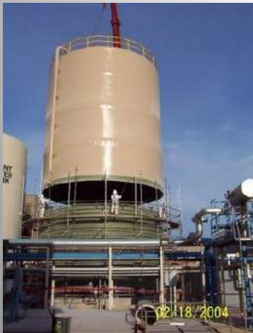
350,000 gal. potable water tank
