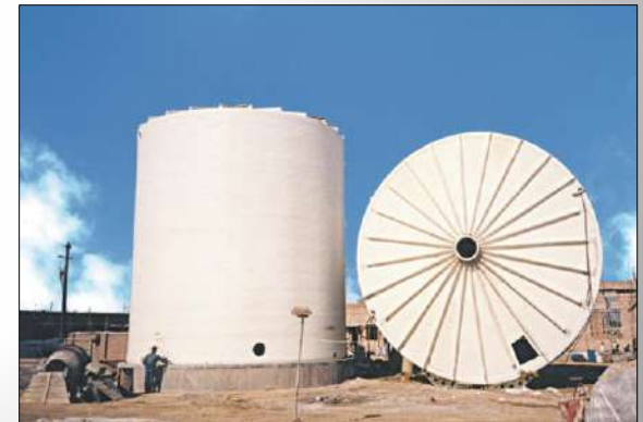
On site tank installation
