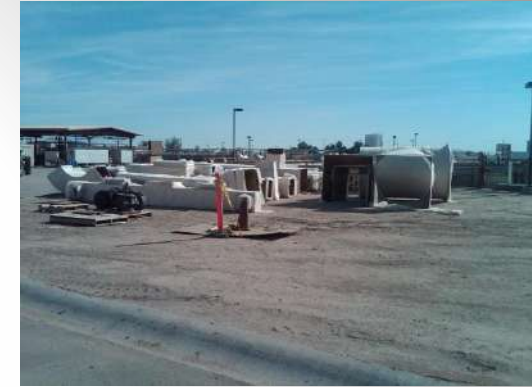
FRP duct for WWTP plant Arizona
