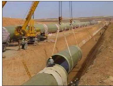
19 km. of 3.1 M water pipe
