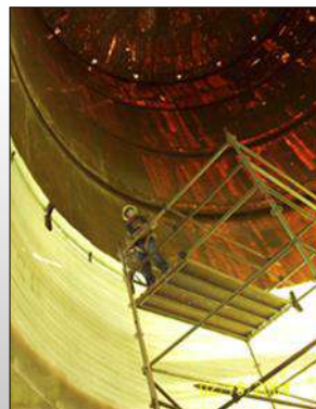
Completed & hydro tested;
