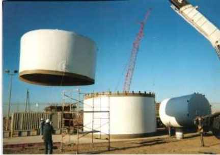
30' dia. x 26' high acid storage, made in Texas, shipped to California
