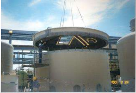
25' dia. x 14' high clarifier, made in Texas shipped to California for assembly
