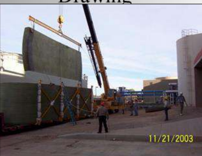
Unloaded on site in Arizona
