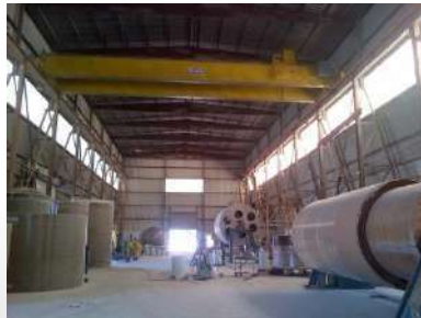
Shop fabricated tanks
