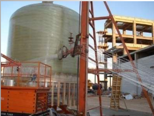
Field winding of large tanks
