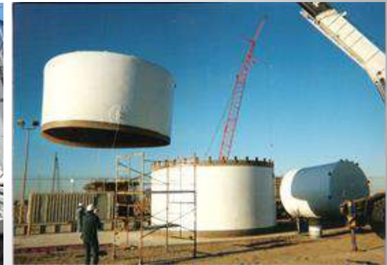
On site tank installation
